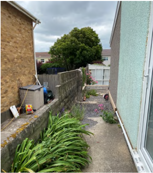
Photograph showing land levels
