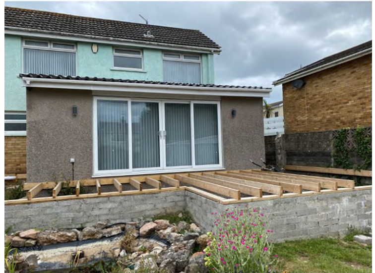
Photograph showing deck in relation to Boundary & No 19 Rest Bay Close
